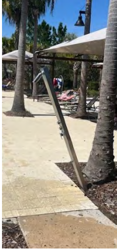
Pool Deck Shower
