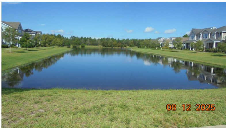
Pond 1b: This pond was in fair condition. The water level is normal.
