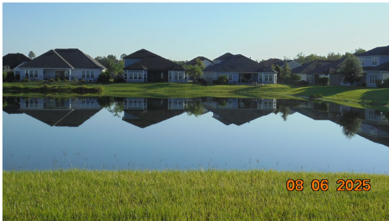
Pond 9b: Pond was in good condition. The water level is normal.
