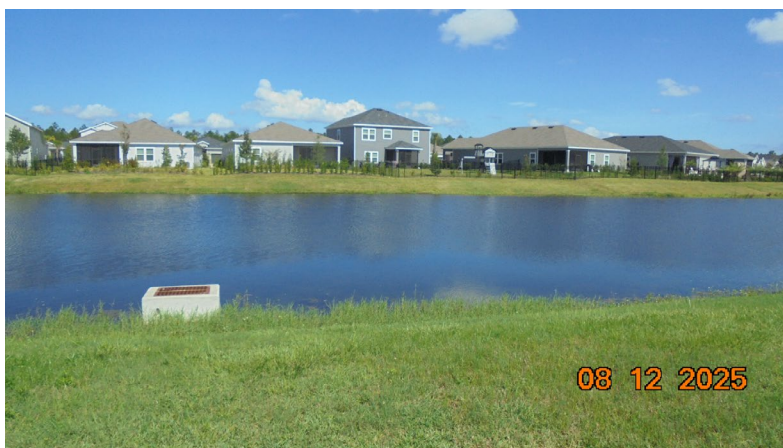
Pond 24c: Pond still under construction.
