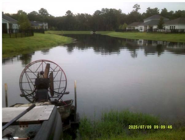
Pond 22B: Pond was in fair to good condition. The water level is good.
