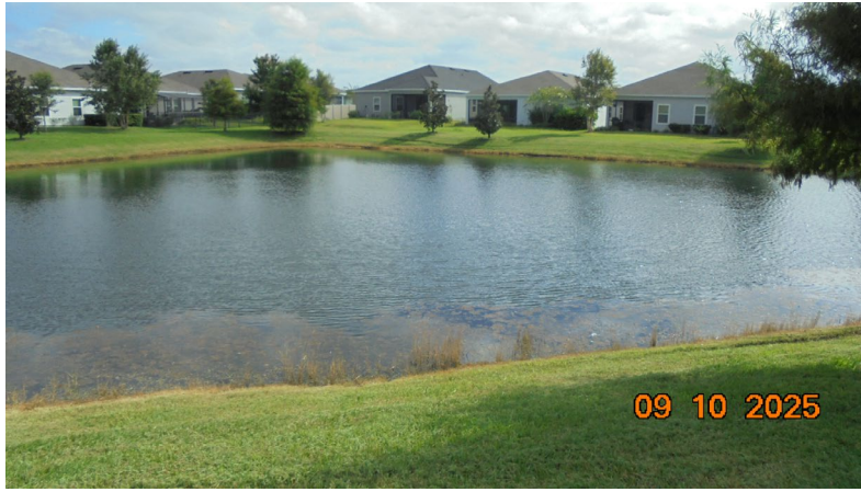
Pond 11b: Pond was in improved condition. The water level is good.
