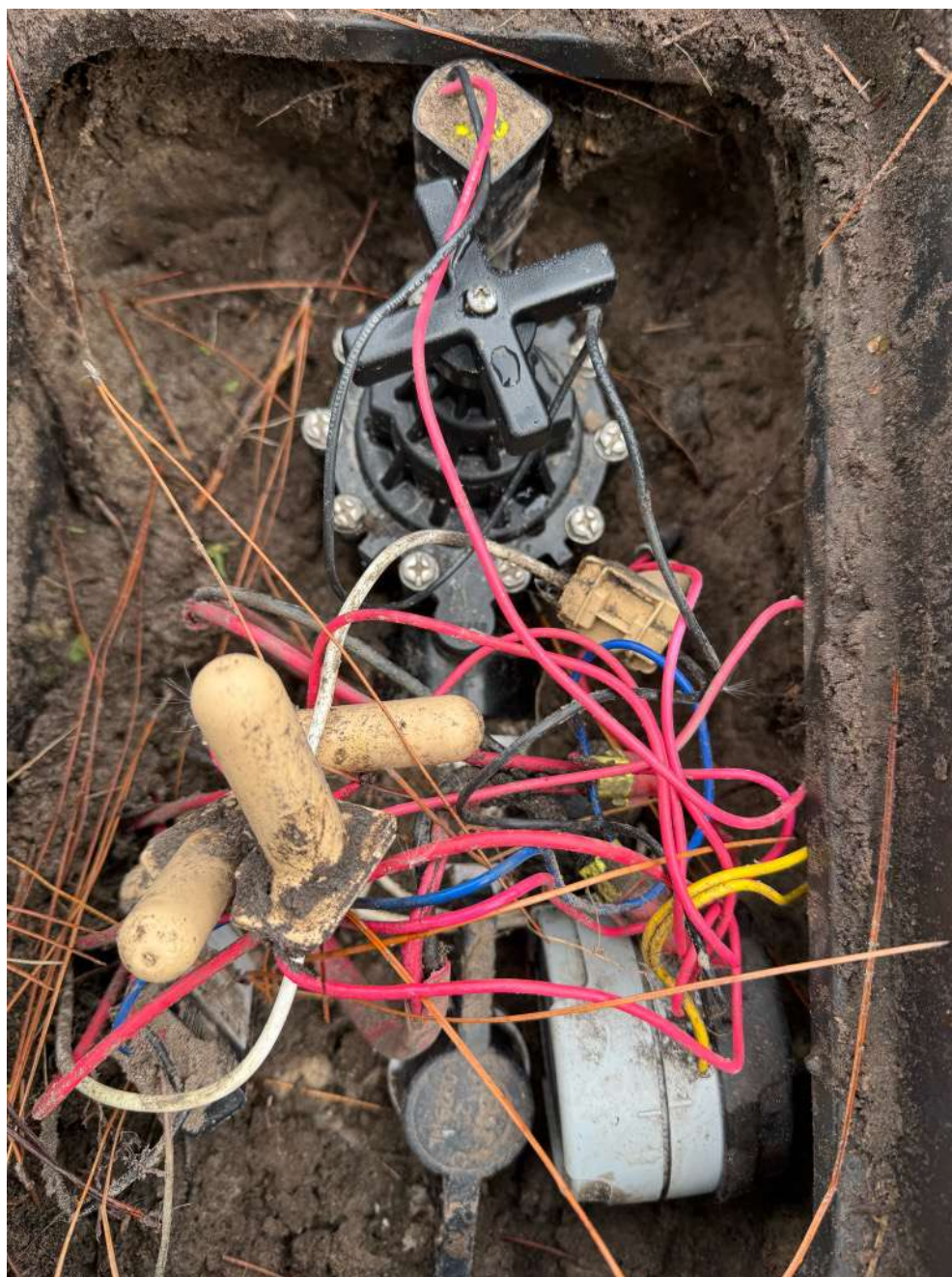
Repaired Broken Irrigation Valve At Rear Of Maintenance Shed
