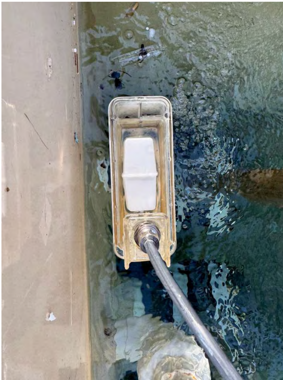
Replaced Fill valve At Lap Pool Surge Tank.
