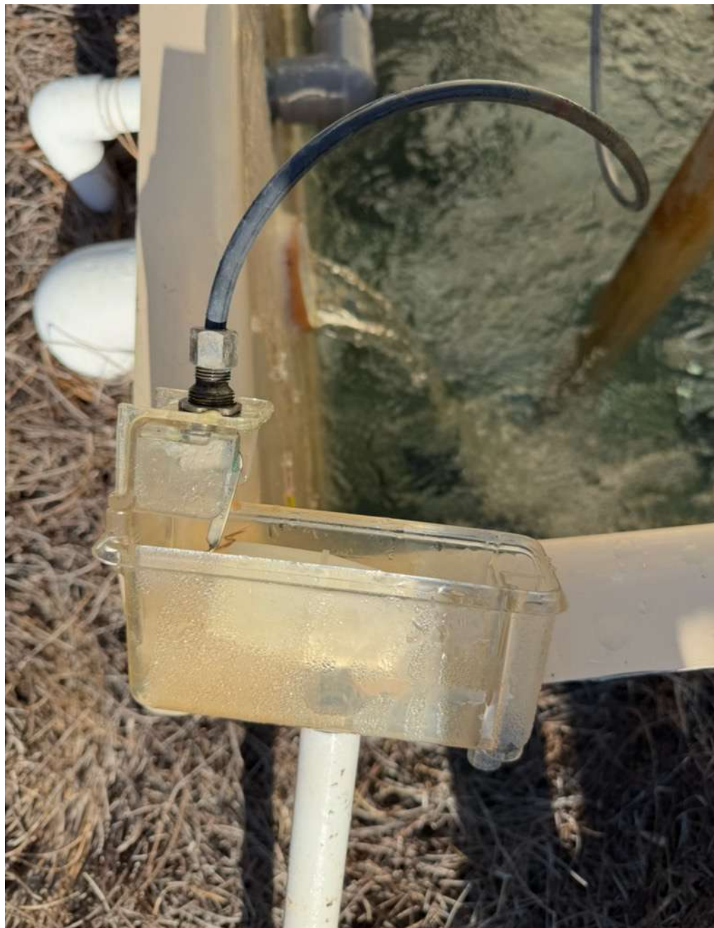
Replaced Fill valve At Lap Pool Surge Tank.
